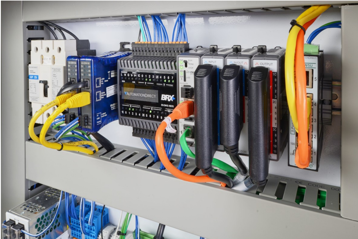
Figure 2: COVER: Next-generation PLCs, like the AutomationDirect BRX Series, are built from the ground up with OT and IT communication protocols, and the necessary security features, for enabling seamless data integration. With the free programming software, users can configure the BRX (with or without classic I/O) to also act as a data gateway. Courtesy: AutomationDirect
