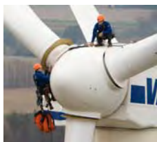
Manual Blade Inspection
