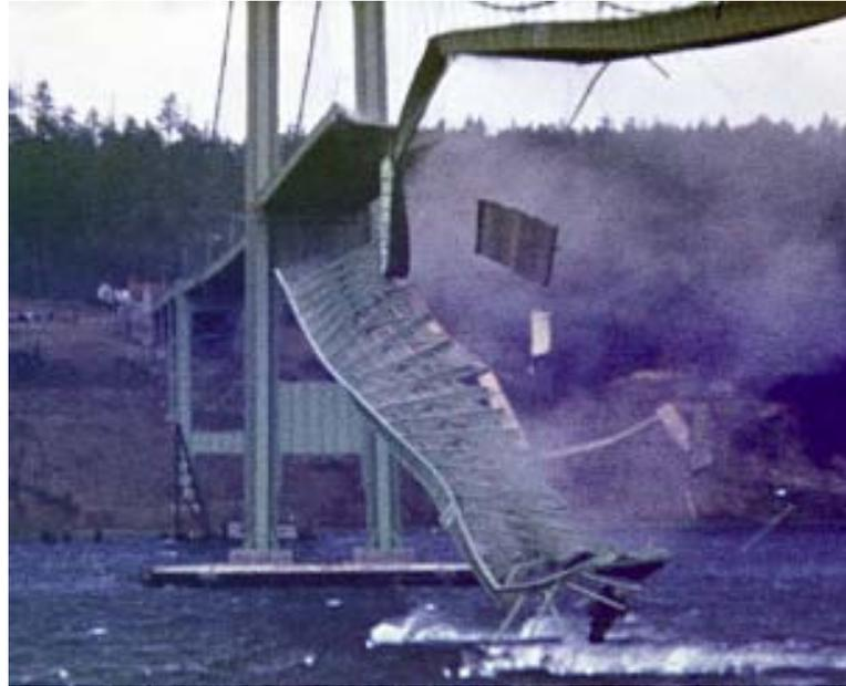
The failure of the bridge occurred due to a never-before-seen twisting mode produced by winds at a mild 40 mph (64 km/h).
